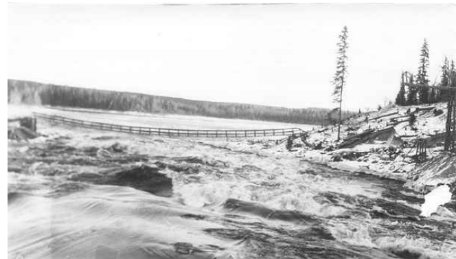
Lower Ear Falls before dam construction 1928.
